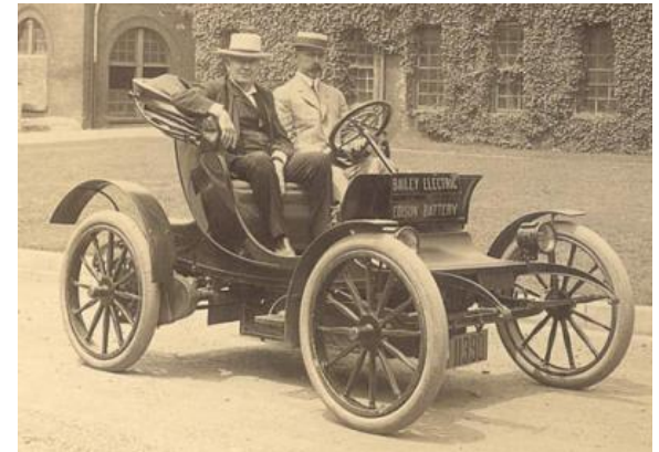
Bailey electric car powered by Edison's NiZn batteries
